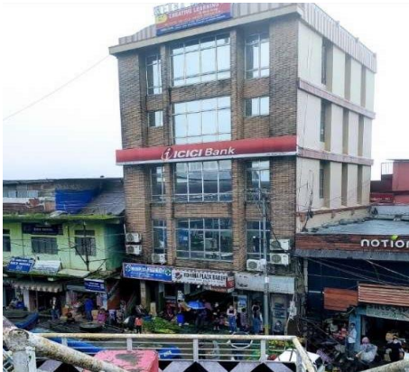
Fig. 8 Buildings of non-uniform Scale along the main street in Kohima
