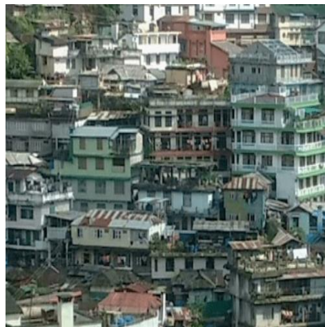
Fig. 13 No open space left within the city due to large built up and high ground coverage
