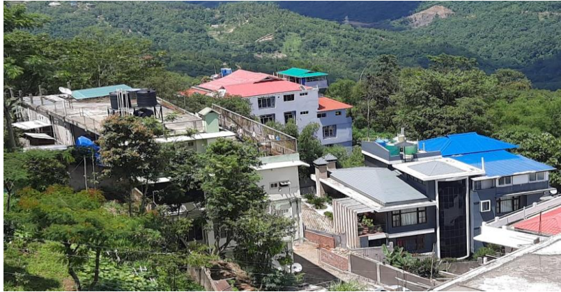
Fig. 2 Buildings being constructed with non-adherence to ground coverage or setback regulations.
